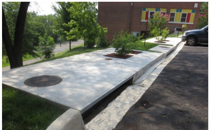
StormGarden with a pre-treatment chamber
